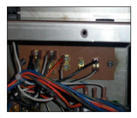
Terminal board inside the heater box
